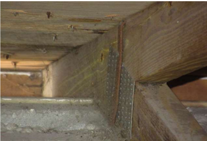
Single strap with 2 nails into the truss
