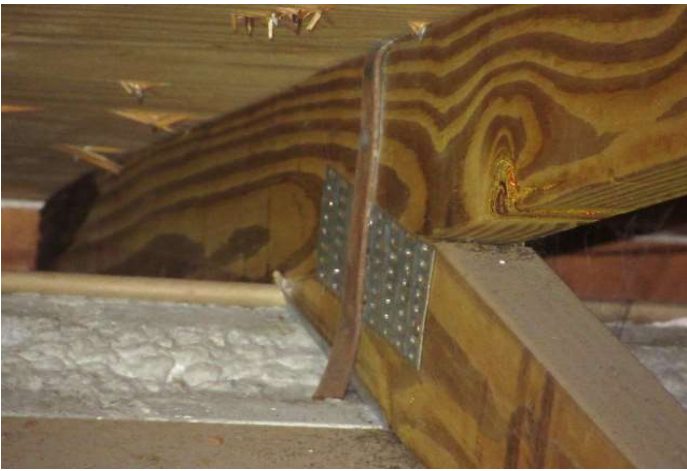
Single strap with 2 nails into the truss
