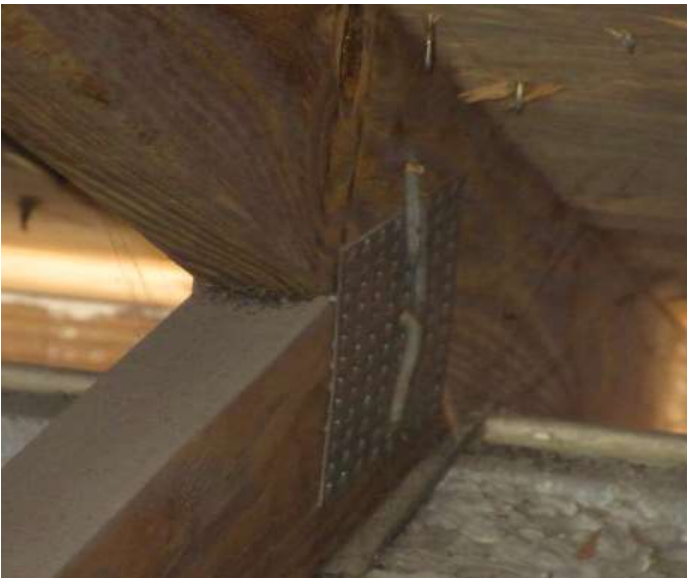
At least 3 nails through the truss
