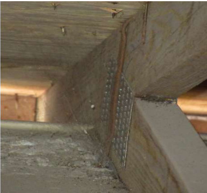
Single strap with at least 3 nails into the truss
