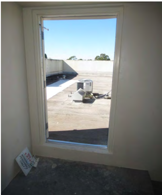
Access onto poured concrete roof
